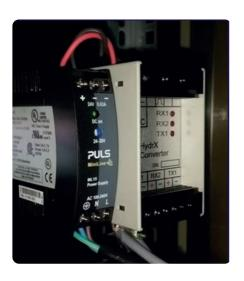
Serial data communication between sensors and instruments is often impossible due to incompatible data protocols. FIELAX developed a programmable converter box solving that problem. It has two input and one output serial RS232/RS422 port (Y-converter). The microcontroller's firmware can be customized e.g. to convert telegrams, merge two input telegrams, resample data or calculate an output from two input ports.
